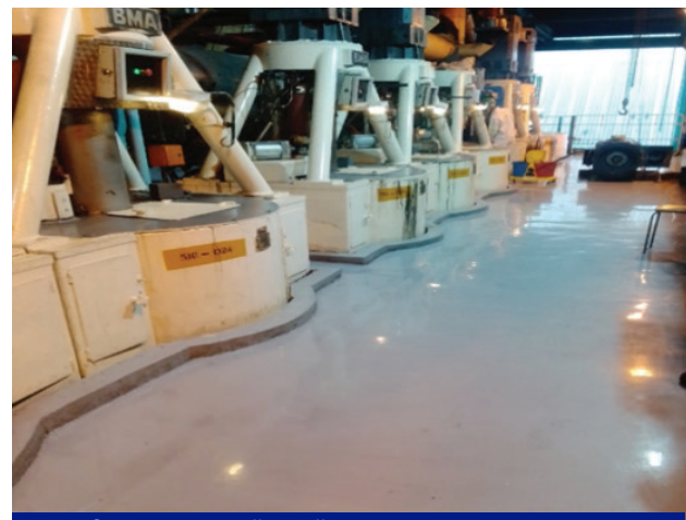
Epoxy floor at Hippo Valley Mill.
