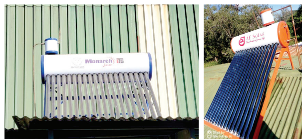
Replacing electric geysers with solar geysers
