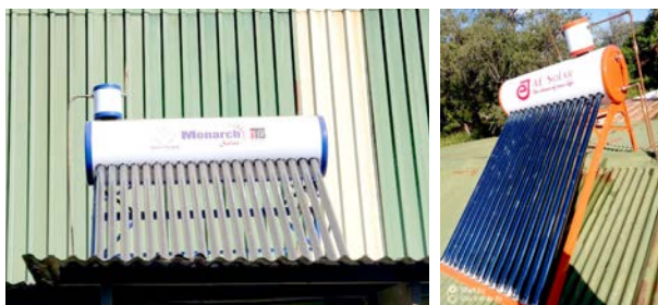
Replacing electric geysers with solar geysers
