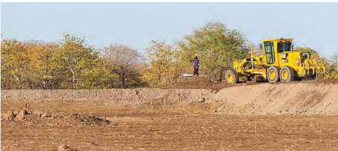
Overnight storage dam construction
